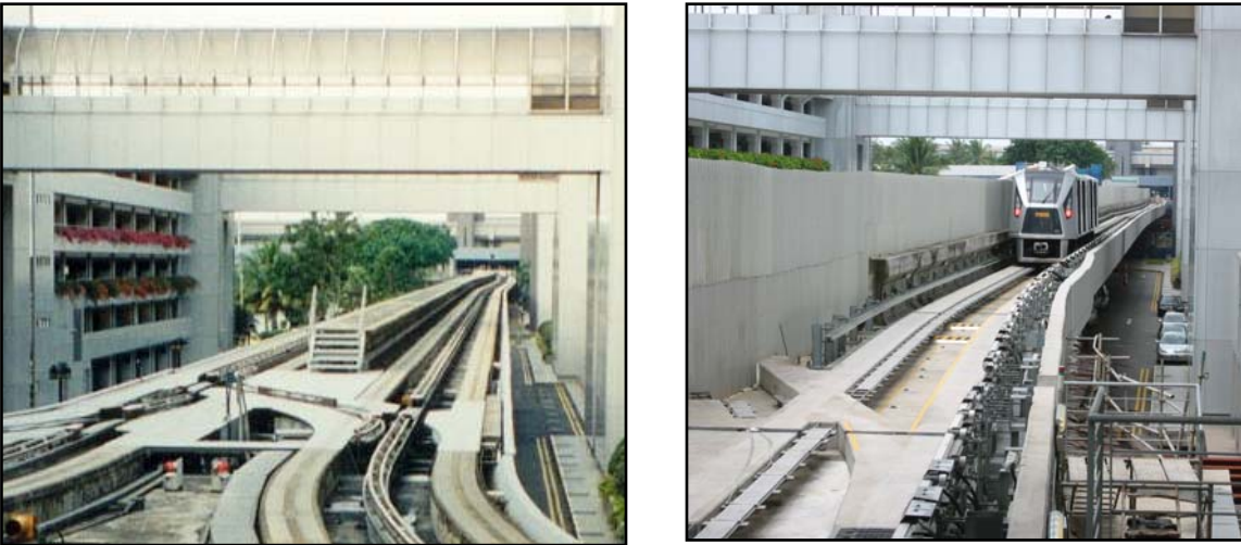
Figure 4. Original and Modified Terminal 1 – 2 Guideway Configurations along Terminal 2.
