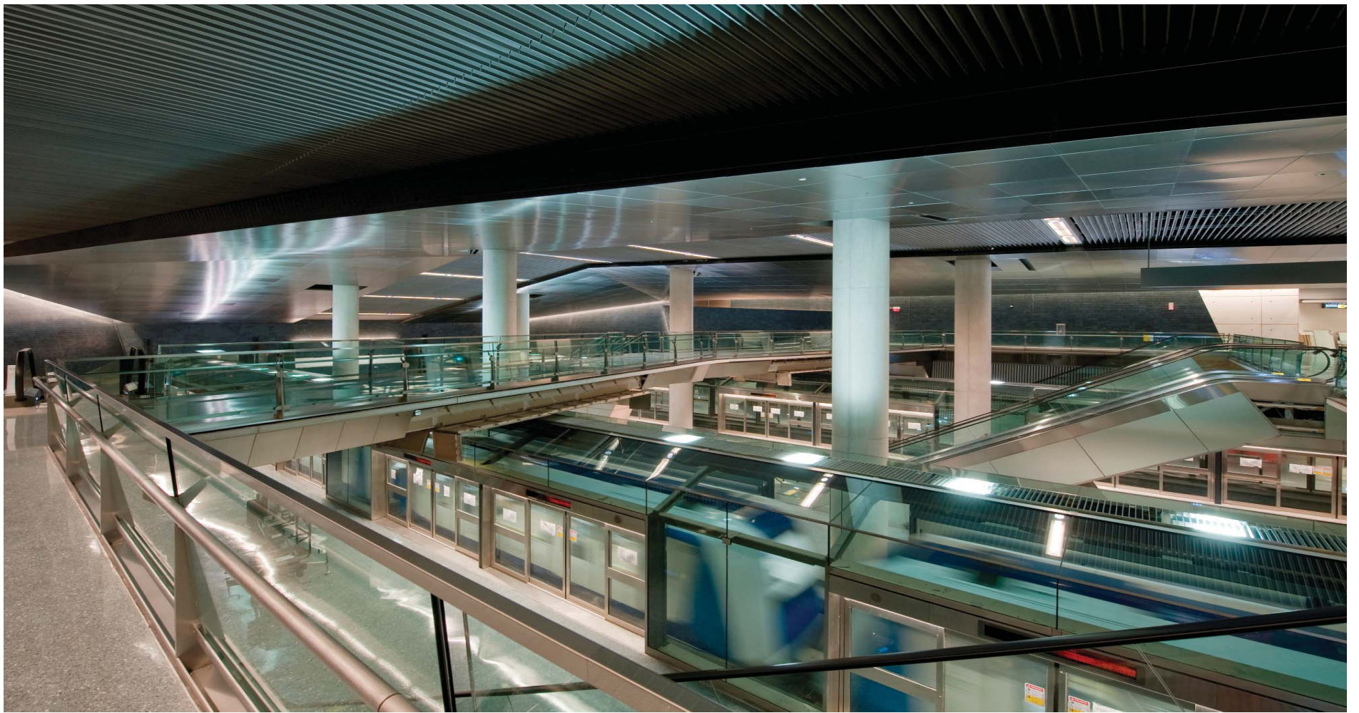
C Gates Station: The AeroTrain station uses side and center platforms.
