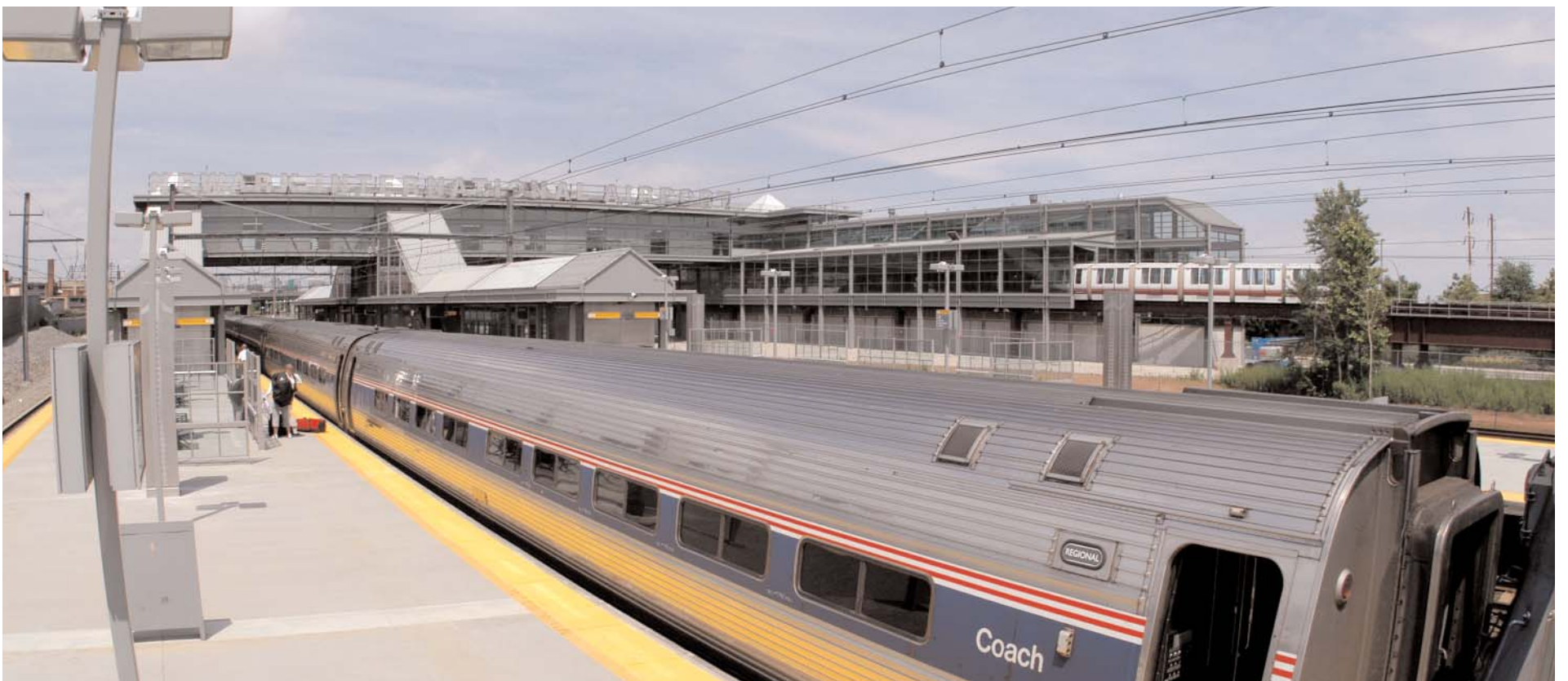
Newark International Airport Train Station provides connection to Amtrak's busy Northeast Corridor and NJ TRANSIT trains.
