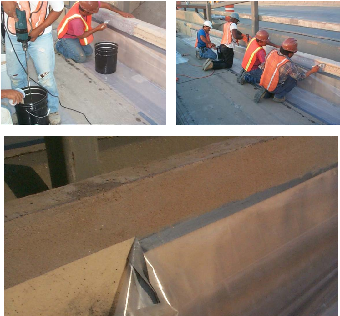
Figure 2: Epoxy-sand grout being applied to parapet wall running surface.
