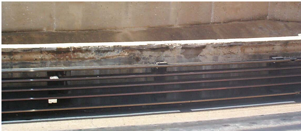
Figure 1: Previous parapet wall running surface repairs.
