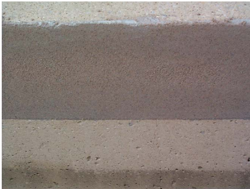
Figure 4: Close-up of epoxy-sand grout repair.
