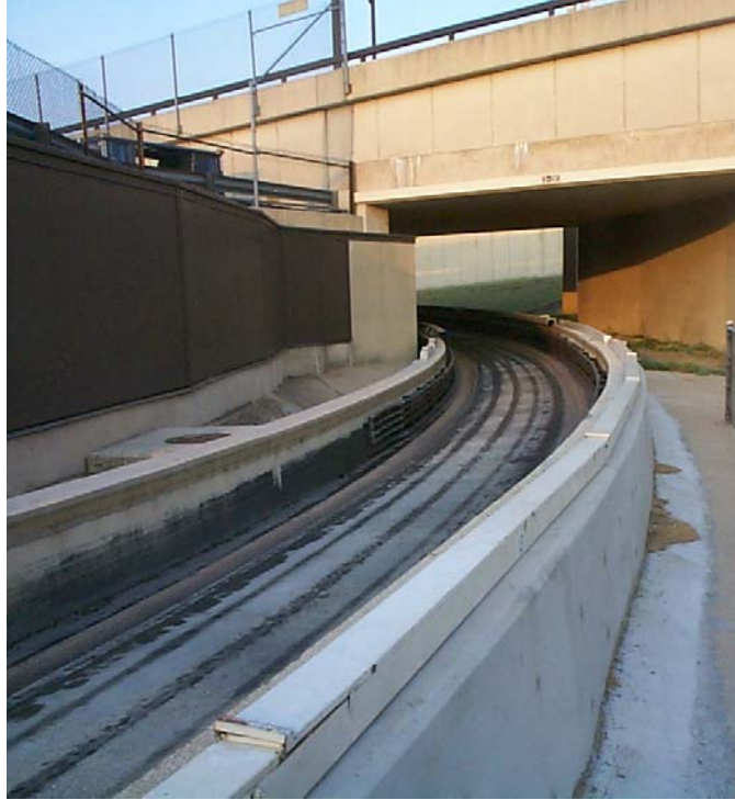
Figure 3: Parapet wall running surface repaired with epoxy-sand grout.
